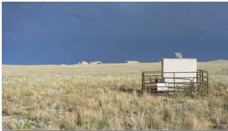
One of the orphaned Spyglass natural-gas wells.
