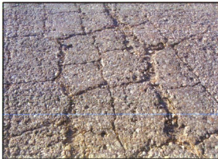
Block Cracking
