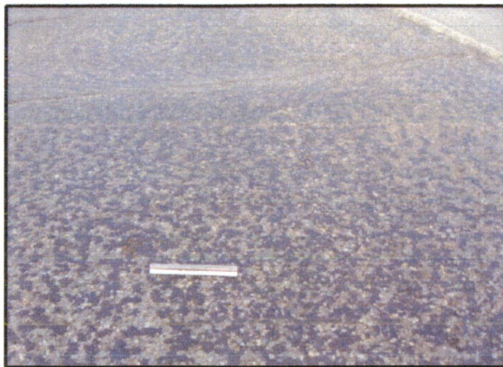
Block Cracking
