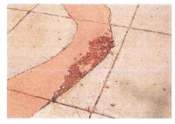
The sidewalk at the Pembina State Museum needs to be replaced. The concrete has broken up in multiple areas and has shifted creating safety issues. The sidewalk repair is estimated to cost \$10,000. In addition, three heat pumps need to be replaced at a cost of \$16,300. The outside lights on the museum are mercury vapor and eventually need to be replaced. We'd like to switch to LED, which will cost approximately \$8,000-\$10,000.
