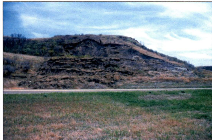
Left: A landslide and broken oil pipeline coincide in Billings County. Right: A landslide to the south of ND Highway 200A west of Washburn. The slope has since been cut back to stabilize it. Whenever possible, the Survey maps areas ahead of development so that infrastructure can be diverted around areas of unstable slopes.
