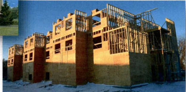
Construction Progress, January 2019
