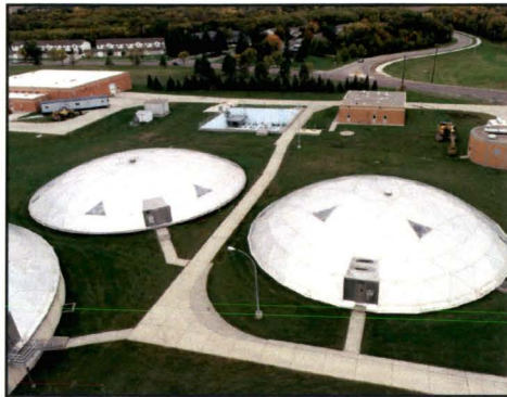
Aerial view of the city of Fargo's Wastewater Treatment Facility (Courtesy of AE2S)
