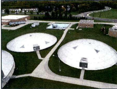
Aerial view of the city of Fargo's Wastewater Treatment Facility (Courtesy of AE2S)
