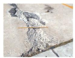
**Pavement deterioration** on Bravo Apron with a yardstick to show scale.
