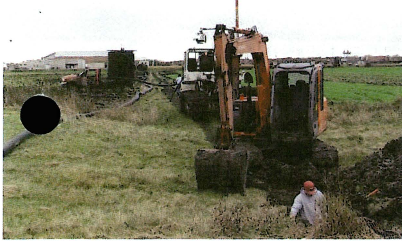
A lot of equipment is required to install tile drainage.
