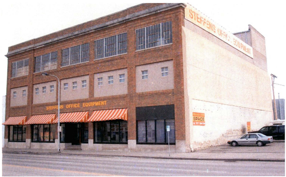
Minneapolis Steel and Machinery, Fargo, North Dakota Before Rehabilitation:
