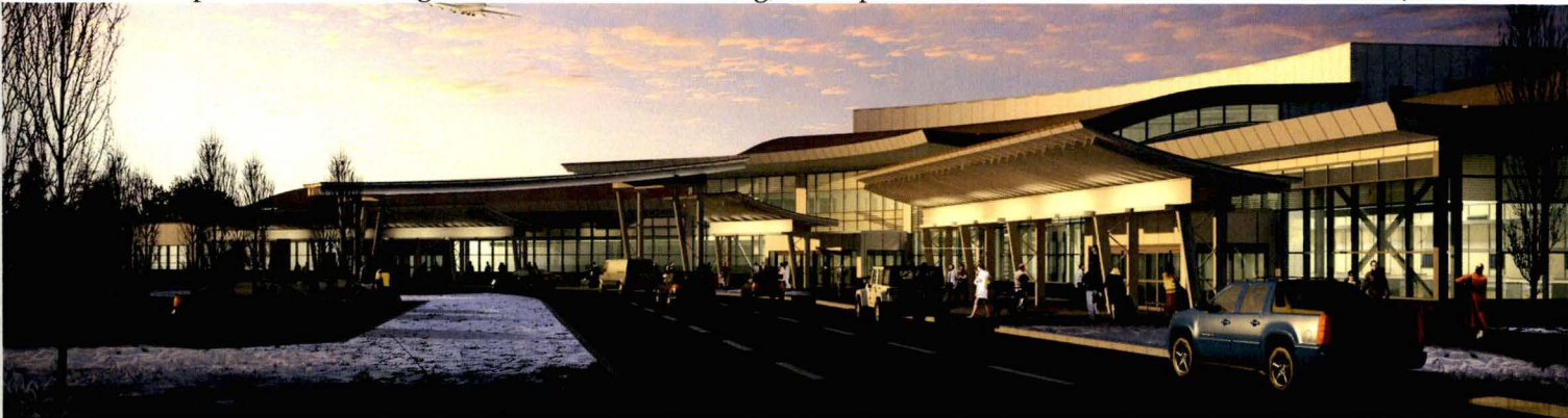
Below: A comparison of the original architectural rendering, and a photo of construction as of December 1st, 2014.
