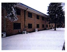
NDVS/SB South Wing. Note multiple split-system air conditioning units. Recommend replacement with centralized system.
