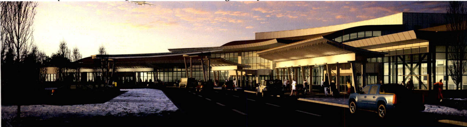
Below: A comparison of the original architectural rendering, and a photo of construction as of December 1st, 2014.
