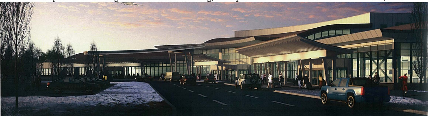
Below: A comparison of the original architectural rendering, and a photo of construction as of December 1st, 2014.
