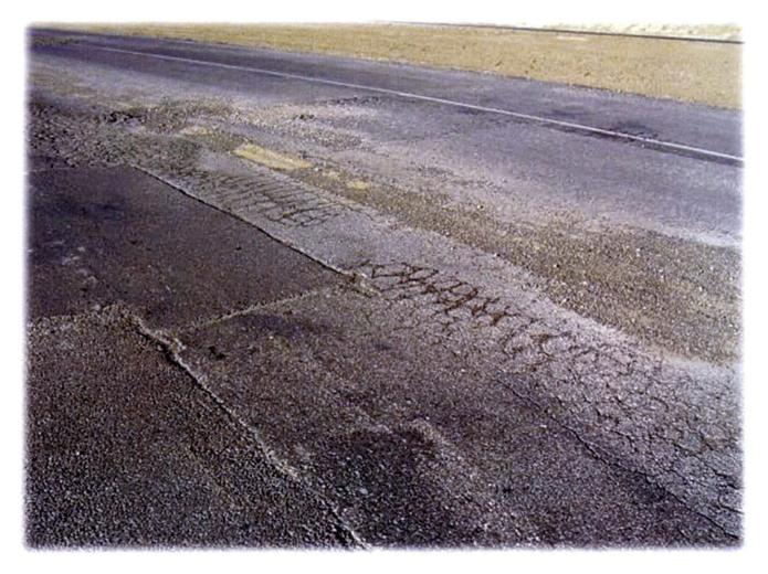
Alligator cracking on ND Highway 23 near Johnson's Corner between Watford City and ND Highway 73.
