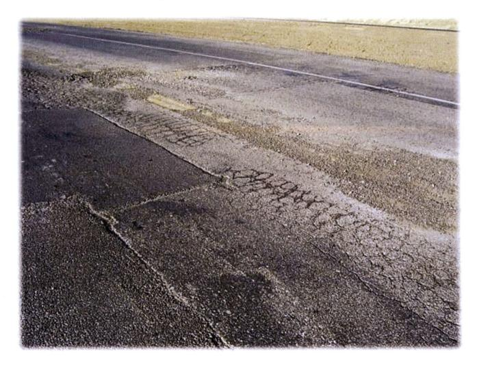
Alligator cracking on ND Highway 23 near Johnson's Corner between Watford City and ND Highway 73.
