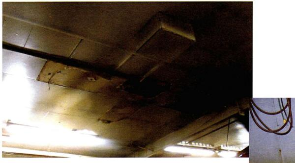
Roof leaking resulted in sheet rock and insulation falling down.
