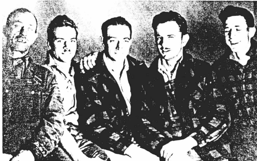
In 1948, these five men were climbing poles and stringing electric lines in the Glendive Division. The line crew consisted of (l to r): Jules Verhasselt, Kermit Parker, Dick Hampton, Frank Pelzer and Gene Poserene.
