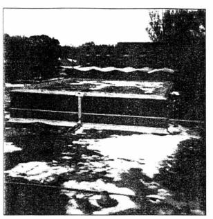
11-5-97 Student Center roof area A-1979, D4-1976 and E-1976. All areas have water leaking into insulation & on decking.
