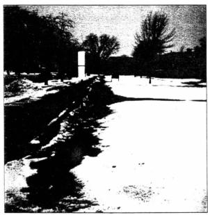
1-30-98 Deteriorated steam lines east of Burch Hall north and south.
