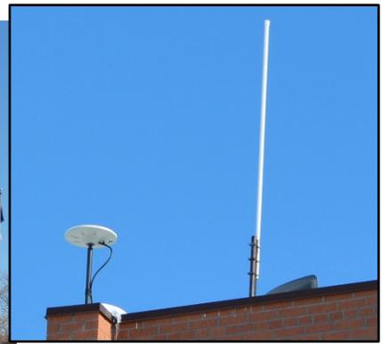
*The GPS base station antennae (a short, cylindrical GPS satellite receiver antenna and a tall, GPS radio signal broadcast antenna) are located on the roof of Schaefer Hall at Bismarck State College.*
