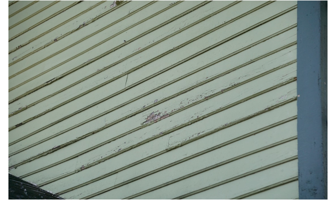
Former Governors' Mansion - Exterior Painting
