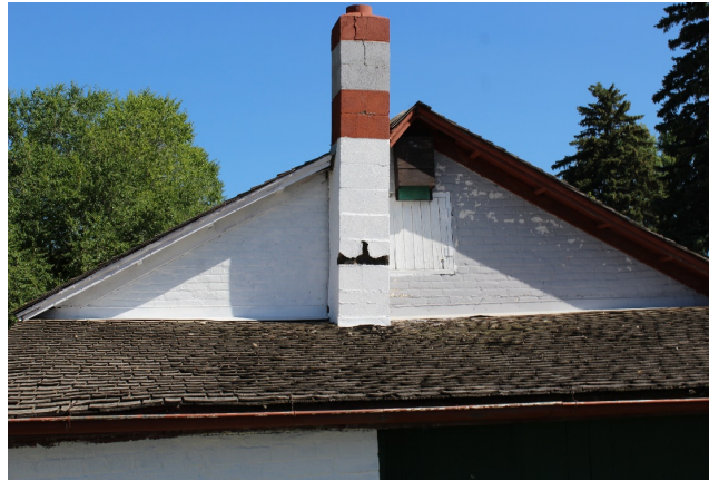
Fort Totten - Shop Chimney Repair
