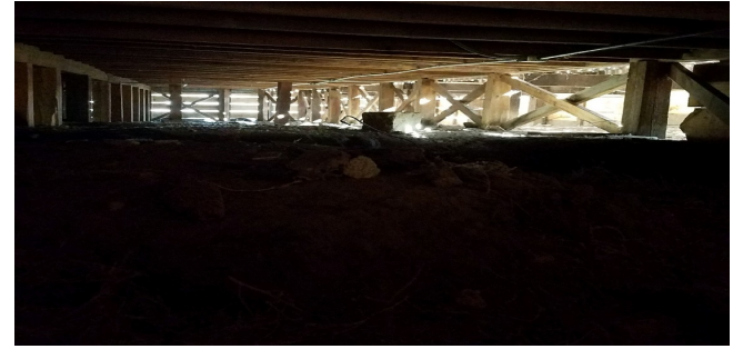
Chateau - Foundation Stabilization
