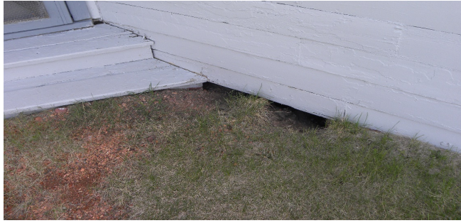
Chateau - Foundation Stabilization
