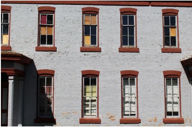
Fort Totten - Girl's Dorm Window Replacement
