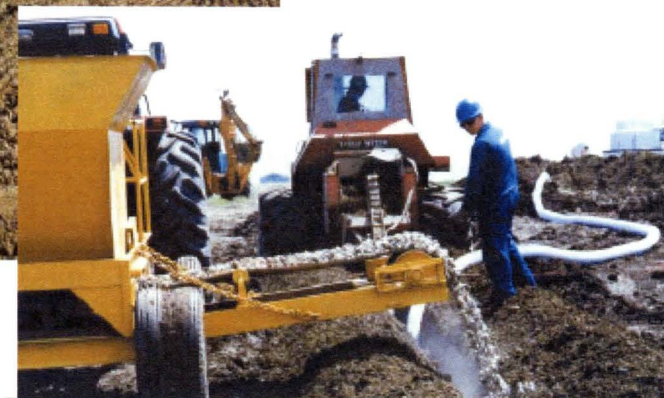
Chain trencher, sock tile, & crushed rock
