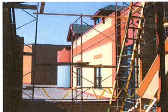
1901 (south) building section: mortar issues in the brick masonry
