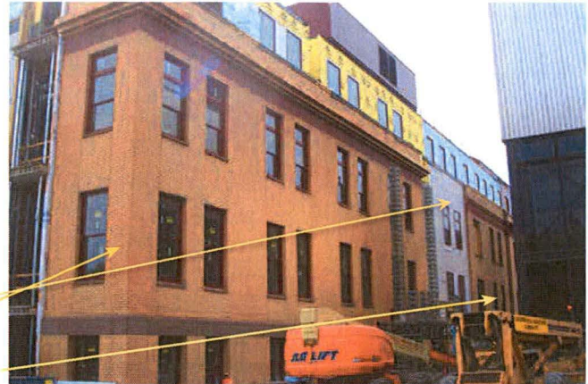
North Addition Rebuilt Collapsed Area 1929 Section
