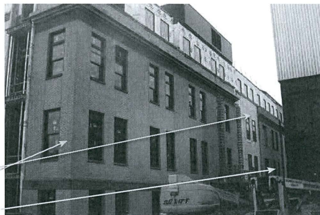
North Addition Rebuilt Collapsed Area 1929 Section
