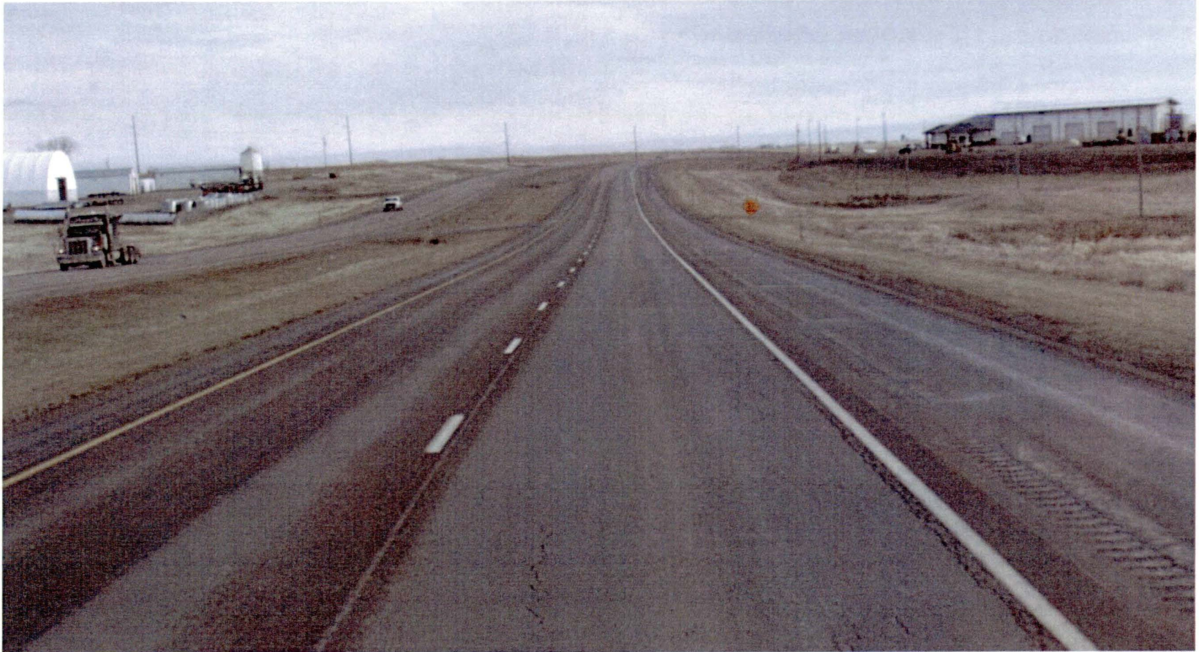
Rutting on US Highway 2 Eastbound Stanley to Palermo.
